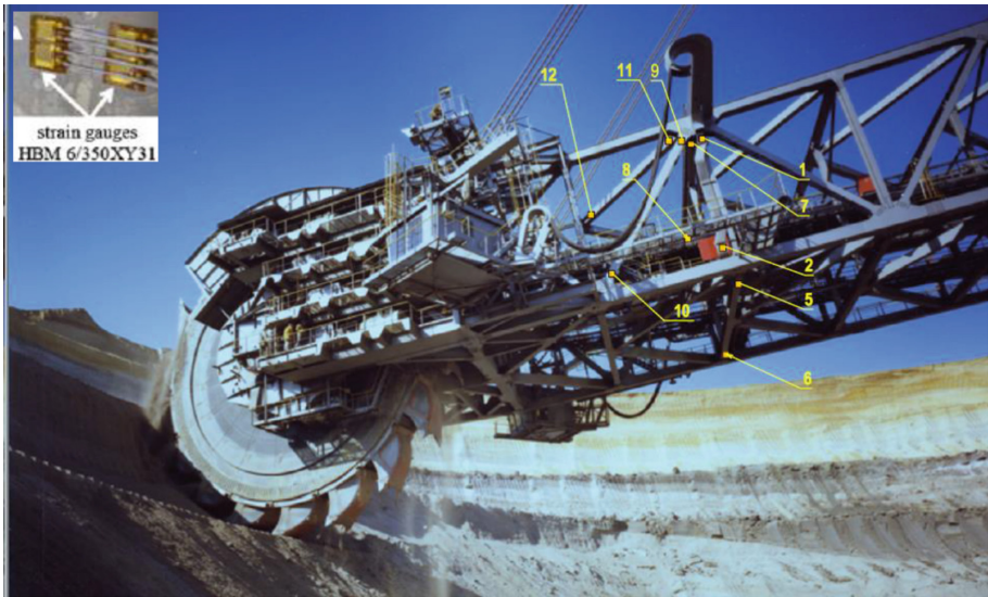
Fig. 2. Placement of the strain gauges on the welded structure of the bucket wheel boom [6].
