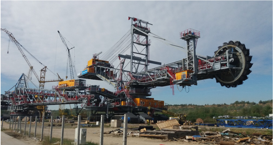
Fig. 10. Bucket wheel excavator Sch Rs 1400 - 28/3 during the assembly, Kostolac (Serbia)
