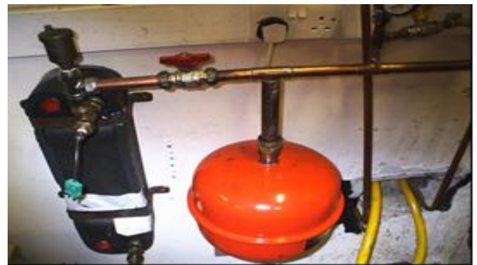
Figure 16. Shows the connections of the heat exchanger and expansion valve.
