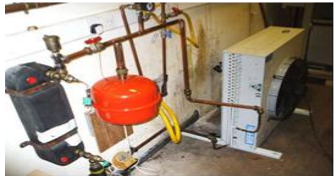
Figure 15. Shows the connections of the heat exchanger, water pump, heat rejection fan and expansion valve.
